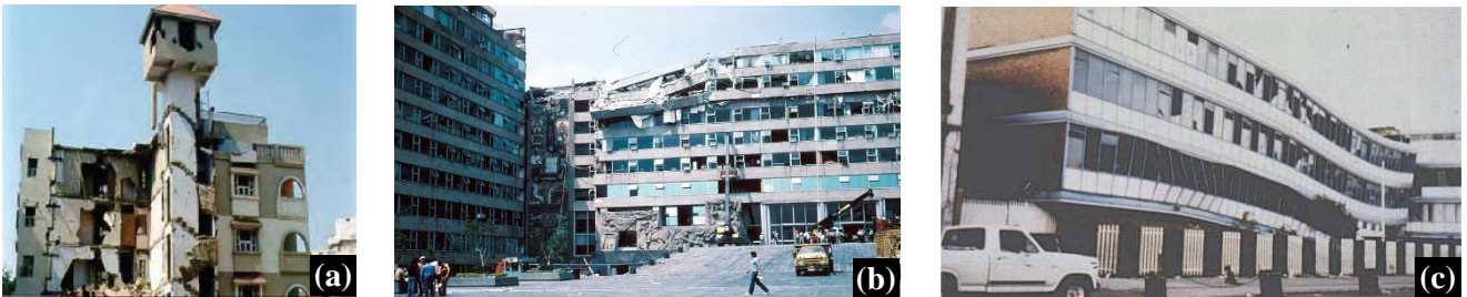
Figure 1: Damage to torsionally flexible buildings owing to: (a) stiff core at center and irregular plan during 2001 Bhuj Earthquake, (b) brittle failure of perimeter columns of upper storeys during 1985 Mexico City Earthquake, and (c) large plan aspect ratio during 1985 Mexico City Earthquake [5-7].
