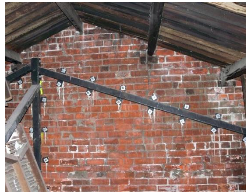
Figure 43: 130 Hereford Street, gable strengthening.
