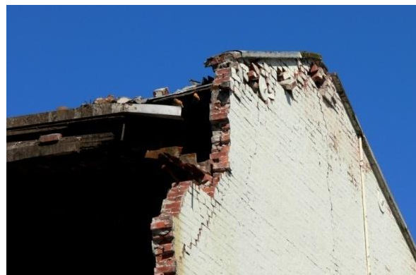
Figure 10: 139 Manchester Street, through steel anchors and rotten timber roof diaphragm.
