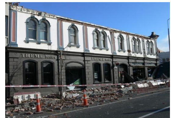
Figure 18: Cecil House / Country Theme Building, 68-76 Manchester Street, concrete beam on the ground.
