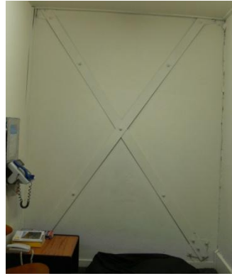
Figure 35: 56 Cathedral Square, 'X' steel brace fixed into wall.
