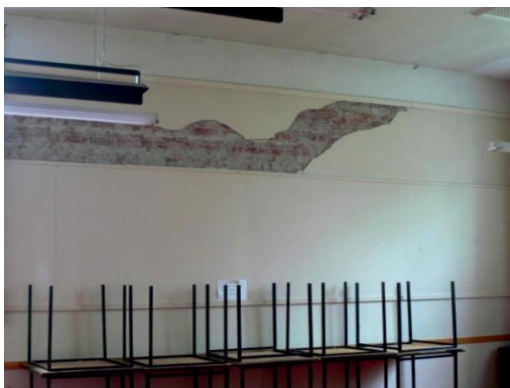
Figure 57: Shirley Community Centre, loss of plaster in north east wall.
