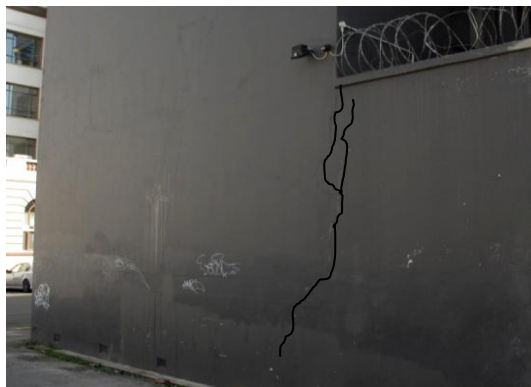
Figure 47: 194 Hereford Street, highlighted crack location at the rear of building.
