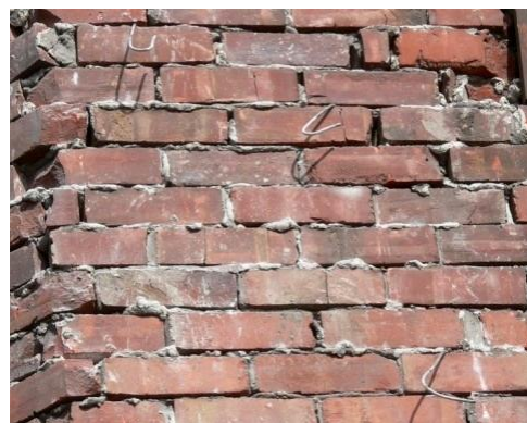
Figure 20: 463-469 Colombo Street, exposed wire veneer ties
