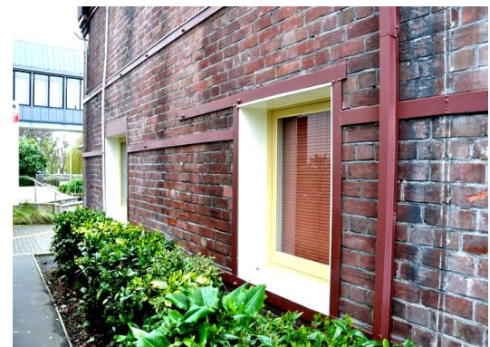
Figure 50: 282-286 Durham Street North, strap detail around openings.
