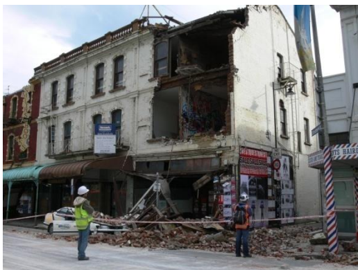
Figure 9: 135-139 Manchester Street, out-of-plane facade collapse.
