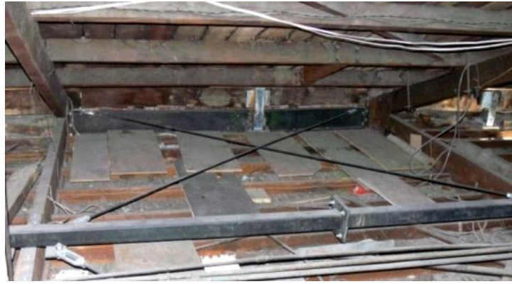
Figure 44: 130 Hereford Street, roof diaphragm strengthening.
