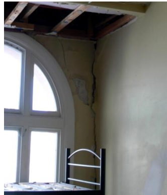
Figure 38: 56 Cathedral Square, façade separation.
