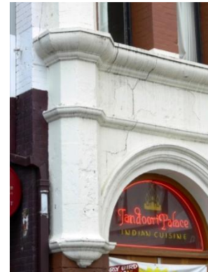
Figure 39: 56 Cathedral Square, cracking through the spandrel on ground level.
