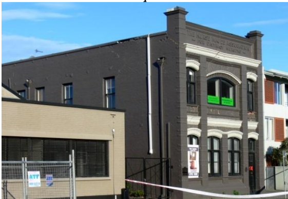
Figure 15: 192 Madras Street, cracking through top spandrel.
