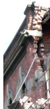
Figure 22: 463-469 Colombo Street, cavity between wall and veneer, with solid parapet above.
