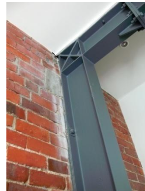
Figure 46: 194 Hereford Street, steel moment frame.
