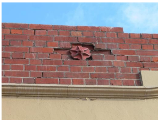
Figure 59: 242 Moorhouse Avenue, wall-diaphragm anchor punching.
