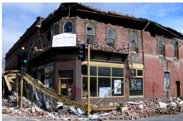
Figure 19: 463-469 Colombo Street, collapse of the veneer.
