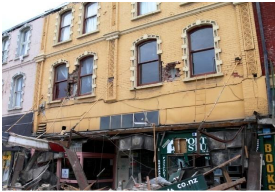
Figure 11: 137 Manchester Street, pull out of the canopy supports.
