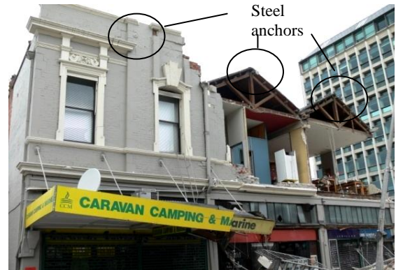
Figure 14: Welstead House, 184-188 Manchester Street, side view, showing steel anchors.
