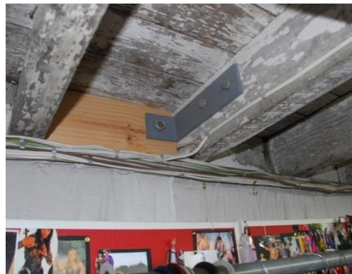
Figure 31: 69-71 Colombo Street, wall to diaphragm connections.
