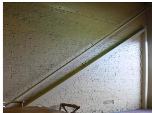
Figure 60: 242 Moorhouse Avenue, wall strengthening using steel sections.
