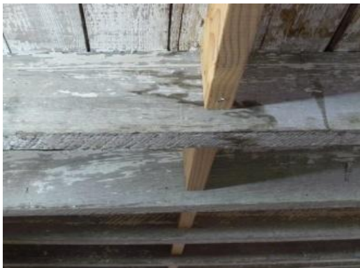
Figure 30: 69-71 Colombo Street, additional blocking at ground floor.
