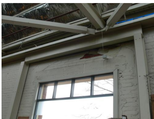
Figure 61: 242 Moorhouse Avenue, interior of the building (location where anchor plate pull out occurred).
