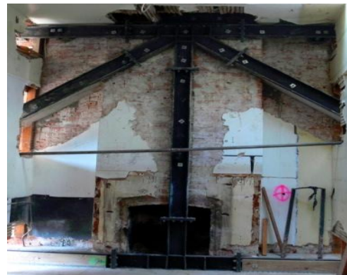
Figure 41: 130 Hereford Street, steel brace frame.
