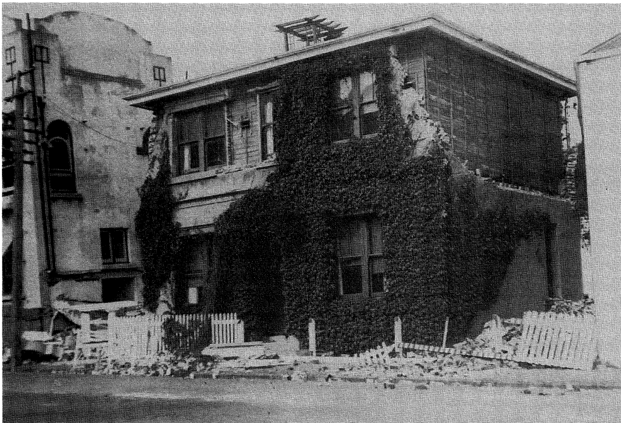
FIGURE 3(C) Example of supposedly Destroyed building: Hawke's Bay Club caretaker's residence, Napier, in the 1931 Hawke's Bay earthquake, stated to be beyond repair (through cracking), but strengthened and still in use in 1996. (Reproduced by courtesy of the Alexander Turnbull Library, Wellington).
