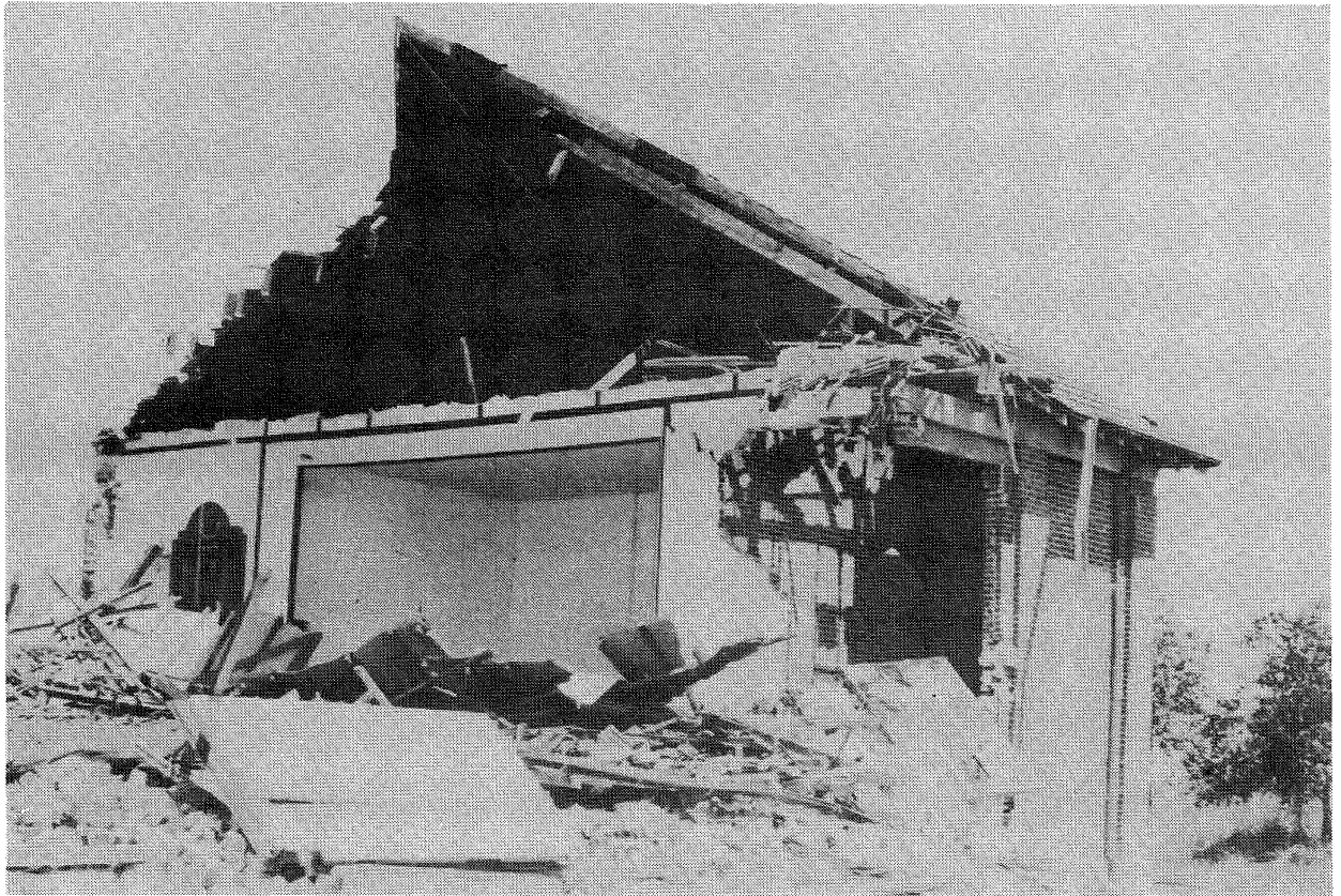
FIGURE 2(A) Example of Collapsed building: Napier Boys High School Assembly Hall in the 1931 Hawke's Bay earthquake, more than 50% volume loss. (Reproduced by courtesy of the Auckland University Architecture Library).
