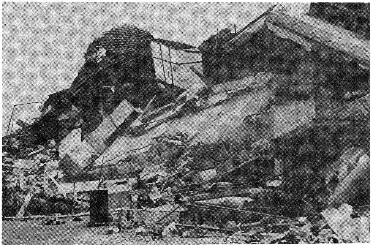
FIGURE 2 (B) Example of Collapsed building: Nurse's Home, Napier Hospital, in the 1931 Hawke's Bay earthquake, 100% volume loss. (Reproduced by courtesy of the Auckland University Architecture Library).
