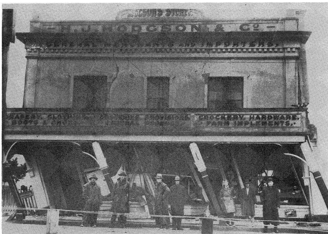
FIGURE 1(B) Example of Partial Collapse: Hodgson's Store, Murchison, in the 1929 Murchison earthquake, small volume loss, not repairable. (Reproduced by courtesy of the Alexander Turnbull Library, Wellington).
