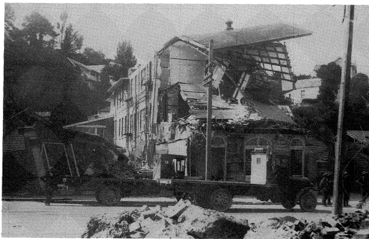
FIGURE 4(B) Example of Partial Collapse: Empire Hotel, Napier, in the 1931 Hawke's Bay earthquake, about 25% volume loss, stated to be beyond repair, but collapsed portion rebuilt. (Reproduced by courtesy of the Alexander Turnbull Library, Wellington).
