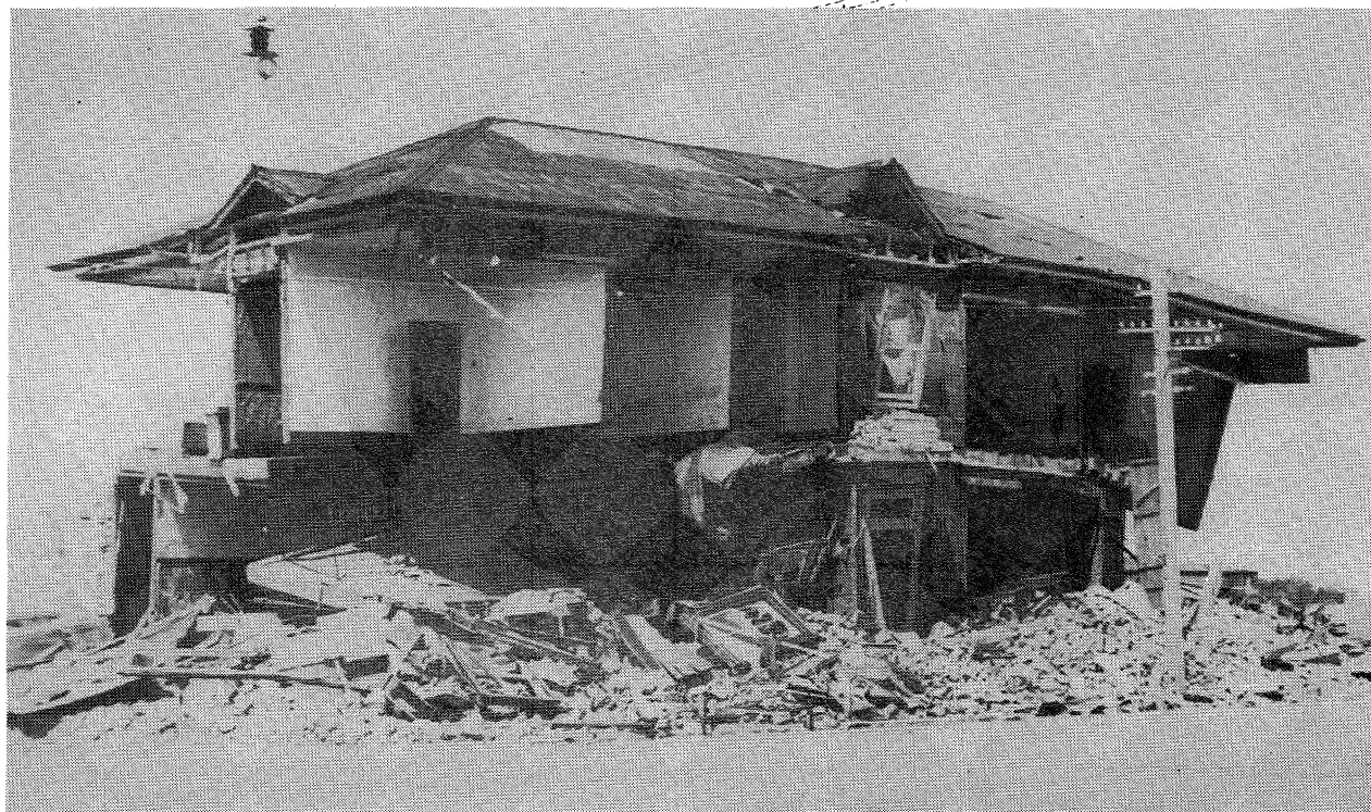
FIGURE 1(A) Examples of Partial Collapse: Taradale Hotel in the 1931 Hawke's Bay earthquake, arguably small volume loss despite collapse of external brick walls, deemed not repairable. (Reproduced by courtesy of the Alexander Turnbull Library, Wellington).
