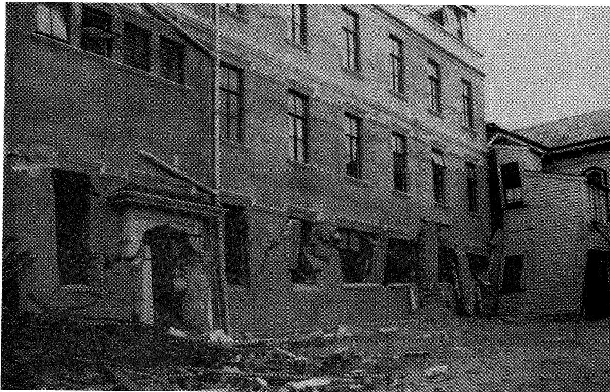
FIGURE 4(A) Examples of Partial Collapse: Seminary at Greenmeadows in the 1931 Hawke's Bay earthquake, small volume loss, stated to be beyond repair, though means of repair were examined. (Reproduced by courtesy of the Alexander Turnbull Library, Wellington).
